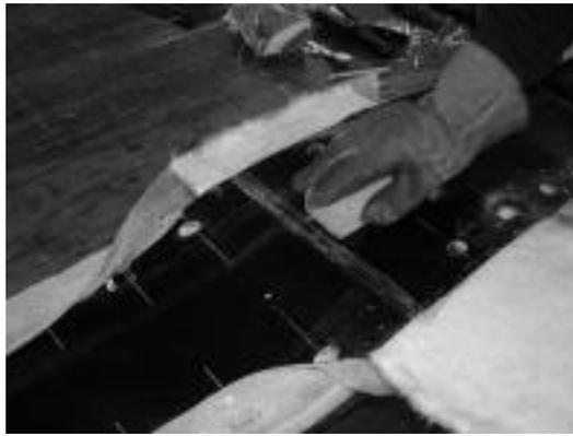
Figure 14 – Press Splice with a wooden block.
