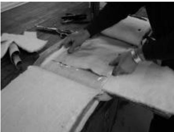
Figure 7 – Position insulation covered plywood board.
