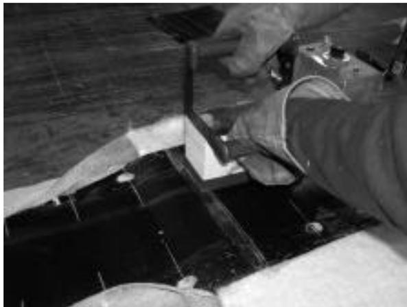
Figure 13 – Position iron and press firmly.
