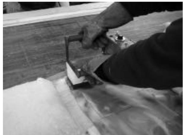
Figure 8 – Position iron and press firmly.
